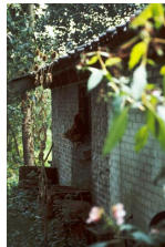
The Cottage, Achterdijk 27, 1988
